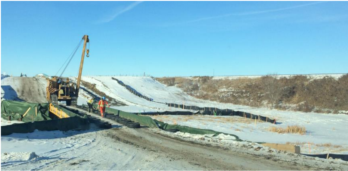
749 + 600 Little pipestone SK WC 87 Creek HER 138 and 139 – Side boom crossing bridge with spotter – pipe strung along right of way and HER sign
