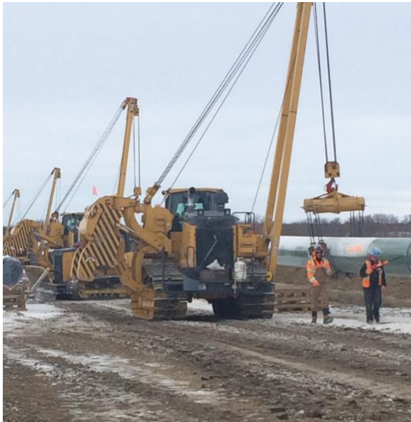
747+300 sidebooms cradle pipe and lowering in ditch with spotters - middle picture below trackhoe shading pipe with spotter
