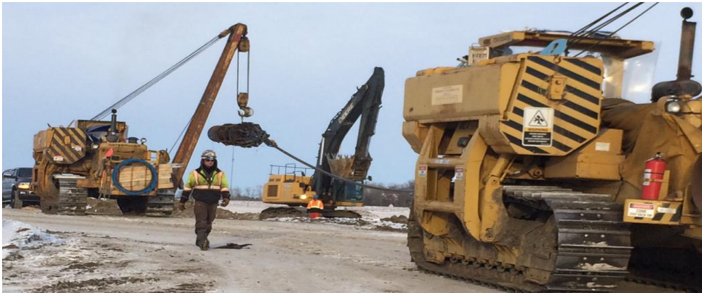
785 + 051 welding crew crossing access
