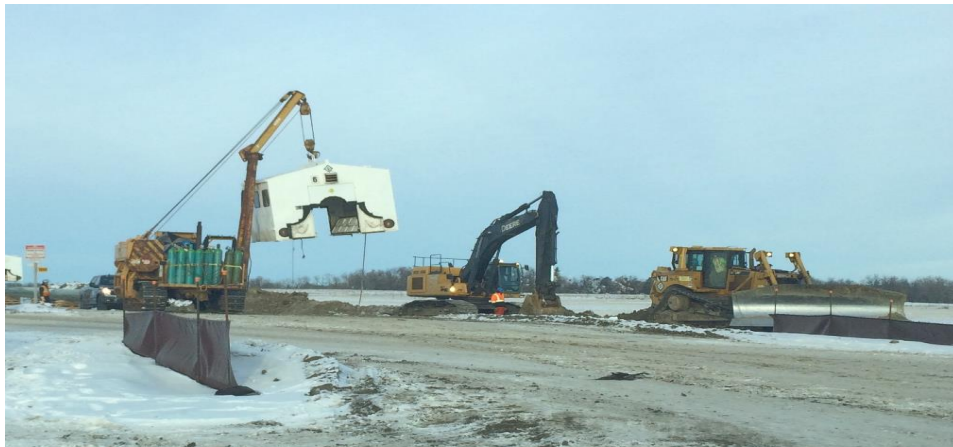
785 + 200 Area of interest roped off pipe strung along right of way
