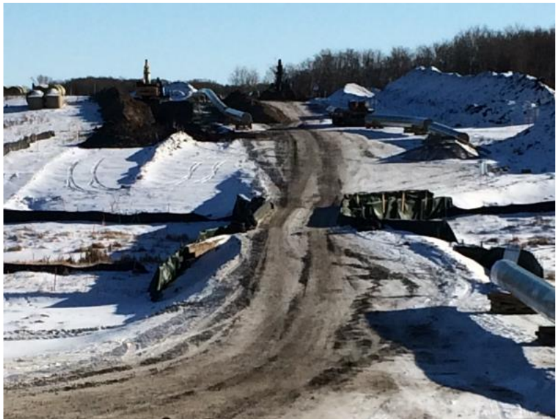
749 + 600 Little pipestone SK WC 87 Creek HER 138 and 139 – Side boom crossing bridge with spotter – pipe strung along right of way and HER sign
