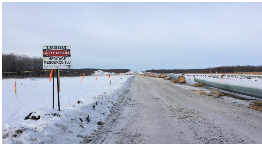
785 + 200 Area of interest roped off pipe strung along right of way
